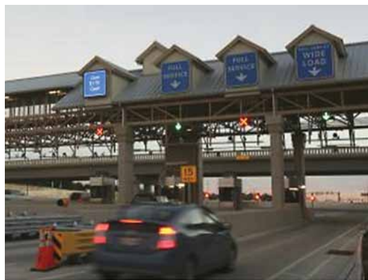
NCHRP Report 689 examines the direct costs of alternative systems of generating revenue, such as this electronic toll collection plaza in Austin, Texas. (Photo: Central Texas Regional Mobility Authority)
