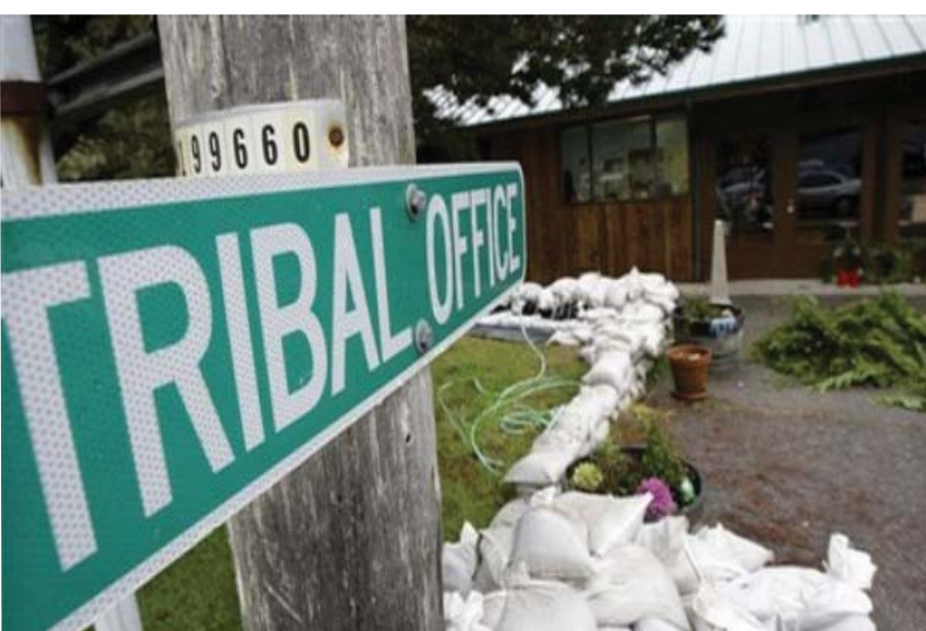
Hoh tribal headquarters are permanently sandbagged due to chronic flooding. (Photo: Elaine Thompson /Associated Press).
