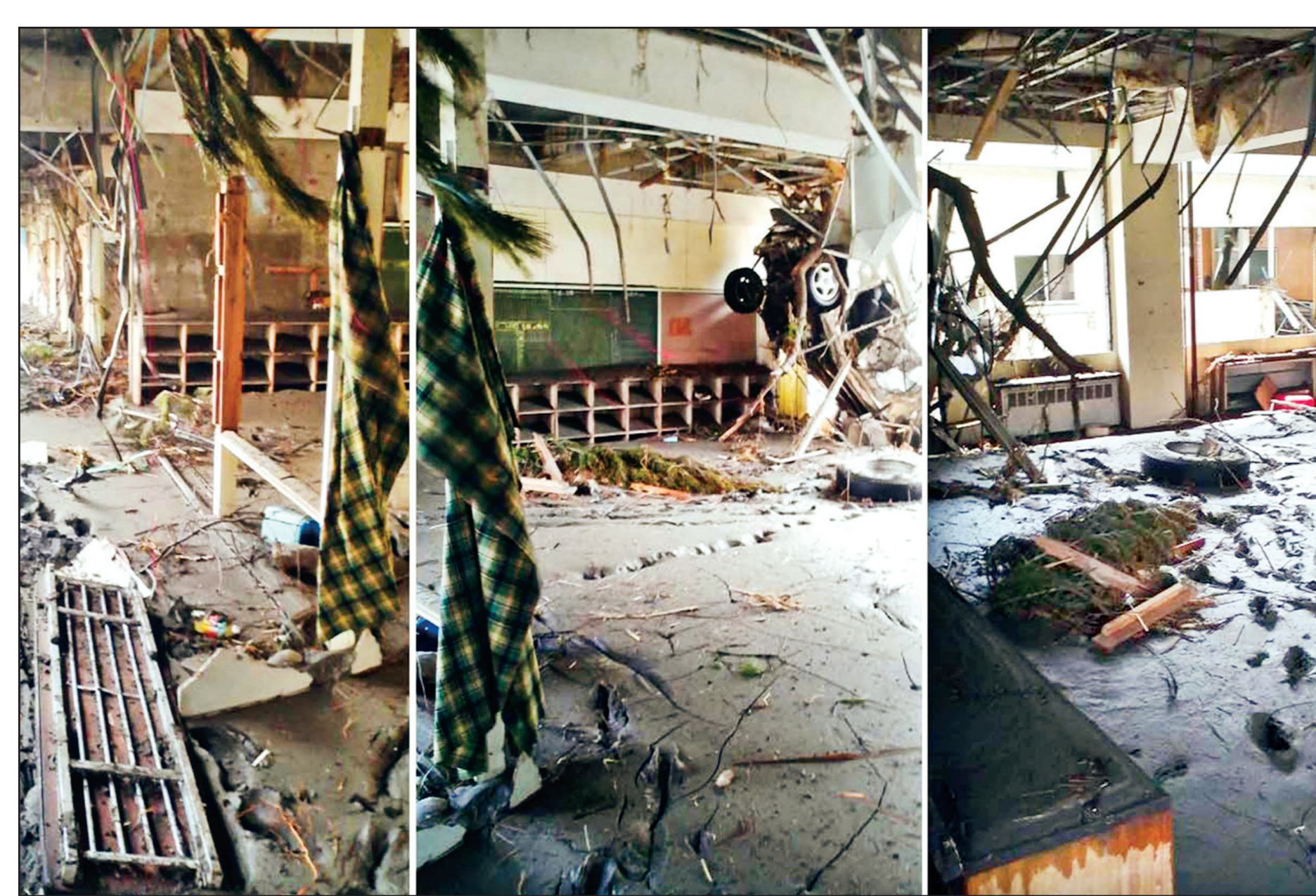
Debris from the tsunami, including a car, litters the third floor of the Kamaishi Junior High School.
