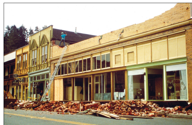
Bricks from the same building fell during the April 1992 earthquake. The building has now been replaced by a wooden structure.
