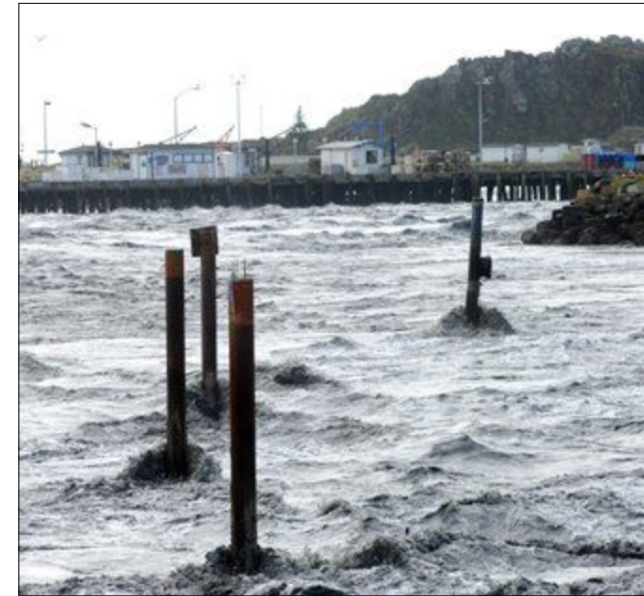
2011 – CRESCENT CITY Strong currents from the Japan tsunami ripped piers apart. It may not look dramatic, but these currents lasted for days and were strong enough to destroy the harbor.
