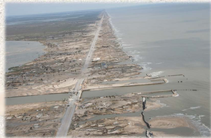
Enhanced building codes allowed one house to remain standing on Bolivar Peninsula, TX after Hurricane Ike. Photo Credit: NOAA
