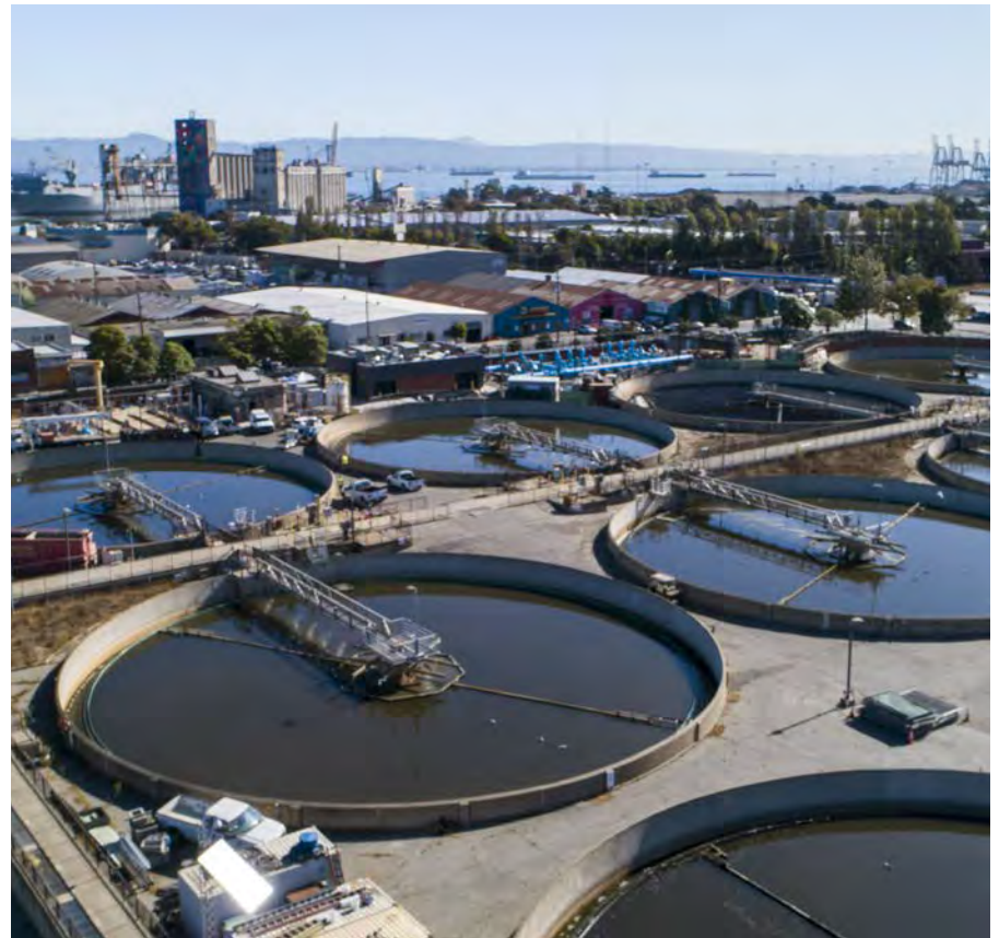
Southeast Treatment Plant
