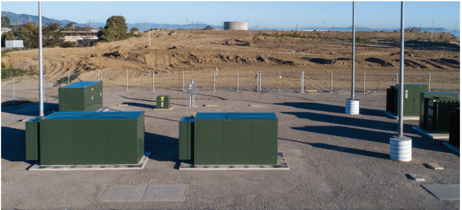
Power infrastructure being installed on Yerba Buena Island
