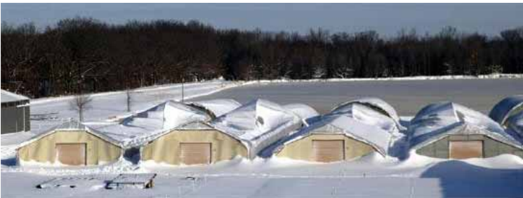
Climate information helps mitigate substantial losses from roof snow loading through structural component design criteria used in about half of the U.S.
