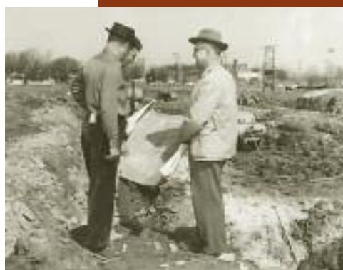
Above: Dean Willard, Gov. Chandler, UK Pres. Dickey and former Pres. Donovan ( top ) at the 1957 groundbreaking for the Chandler Medical Center ( center ). Medical Center construction, 1958 ( bottom ).
