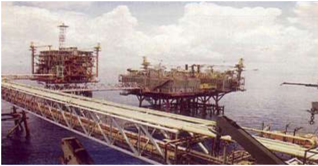
Bach Ho oil exploitation
