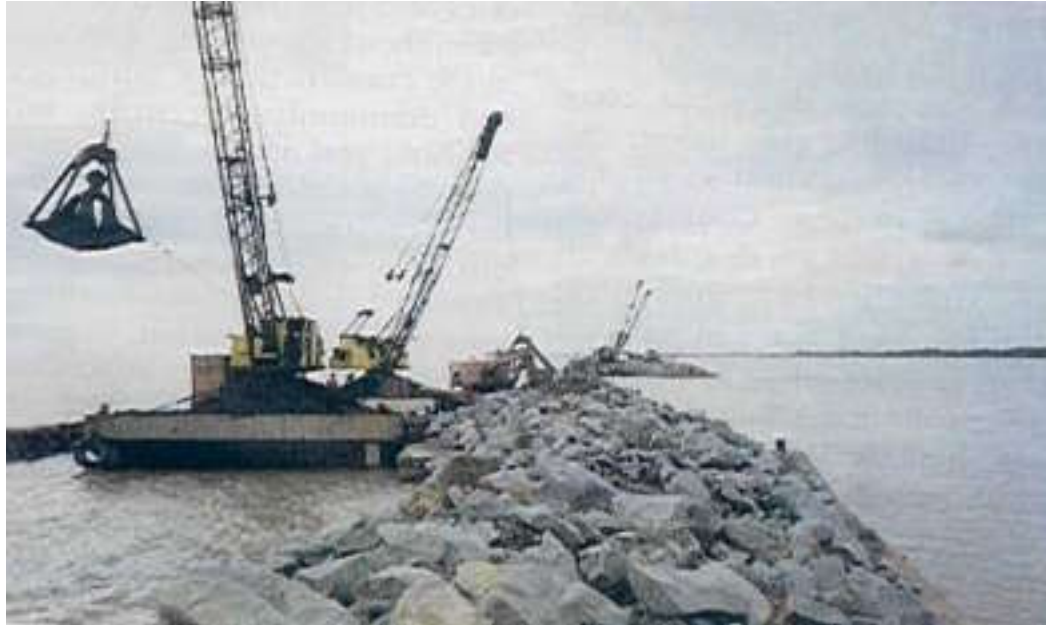
Sea Dyke embankment
