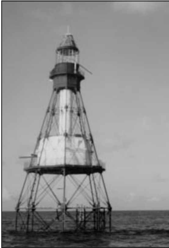
Fowey Rocks C-MAN station before Hurricane Andrew.
