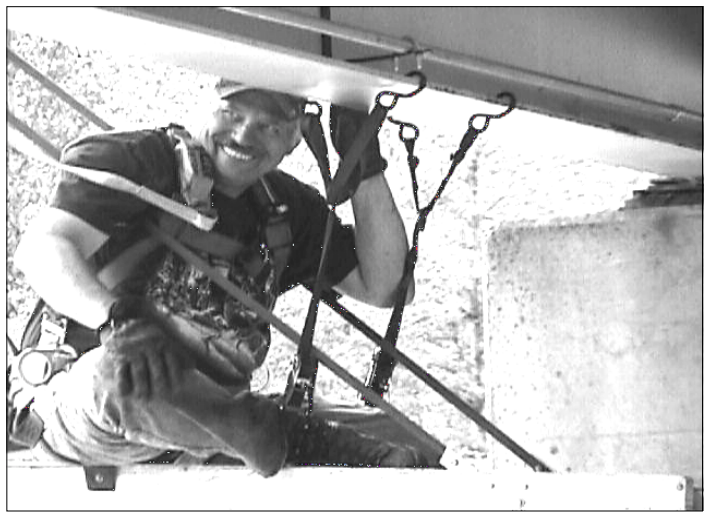
Anchorage Electronics Technicians Dave White (pictured) and Jocelyn Perry installed a depth sensor on the Chilkat River bridge to measure water levels.
