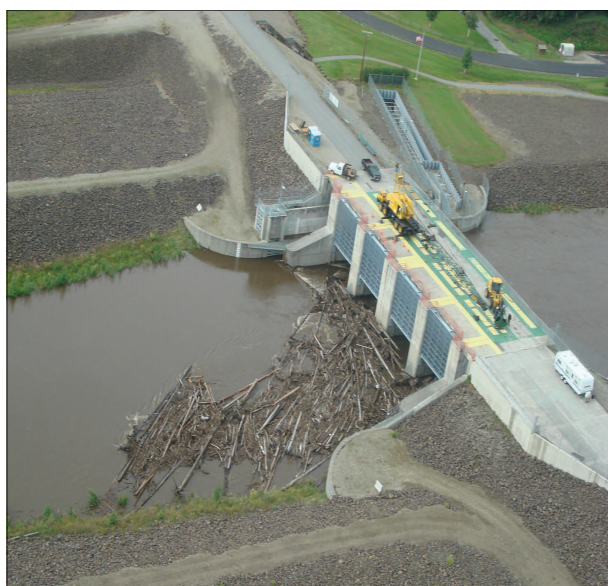
Debris backed up behind the Chena Flood Control Project. The Army Corps of Engineers operated the dam and controlled the flow of the Chena River for approximately 24 hours. Photo courtesy of Ed Plumb
