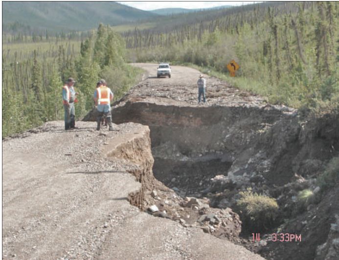
Taylor Highway at Milepost 81, near Walker Fork Campground A culvert washed out, leaving a hole approximately 20 feet deep and 60 feet wide
