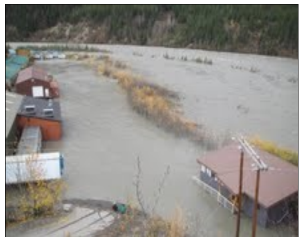
Flooding from the Nenana River near the Denali Park employee housing
