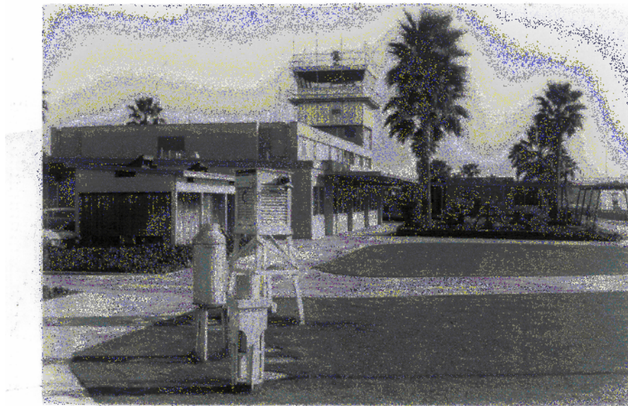
Figure 4 – Weather instruments at Bakersfield in early 1958. A cotton region shelter can be noted in the center of this photograph (Photo courtesy NCDC).
