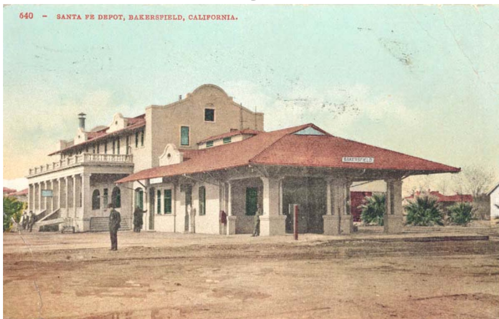
Figure 1 – The Santa Fe Rail Depot in Bakersfield (courtesy Kern County Library).
