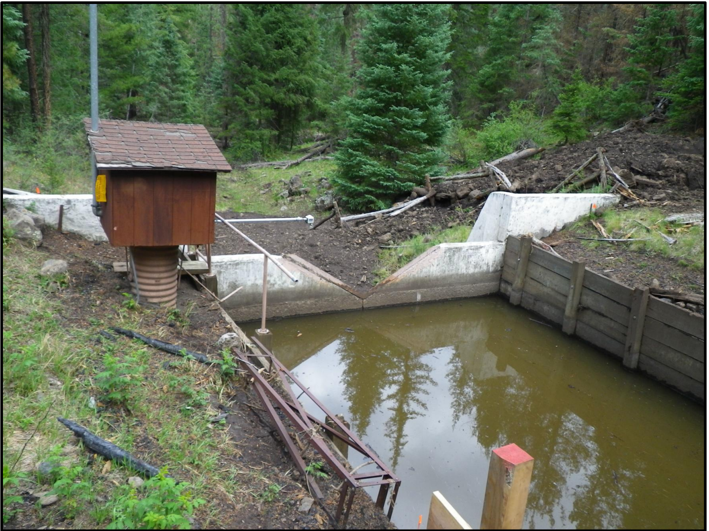
Figure 58. North Fork Thomas Creek Looking Downstream at Weir (photo provided by USFS). From High Water Marks July 11 Flow was 186 cfs +/- 10% at Weir (flow depth was 1.64 feet).
