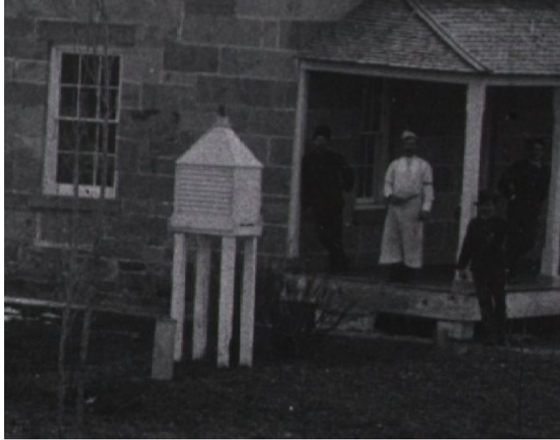
Figure 4. Close up of the cotton region shelter and rain gauge next to the post hospital. Date of Photograph: 1880 to 1895. Source: The History of Medicine (NLM), No. A01048.
