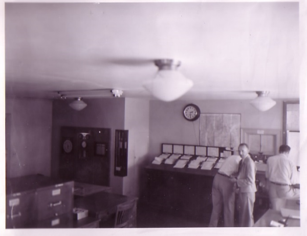
Figure 35. Southeast corner of the observation room at the Boise Airport office. In the photo left to right, the instrument panel, barometer case and sequence table (next to David Stevlingson). Date: 27 September 1950. Source: National Weather Service Boise, Idaho Archives, SL-124.
