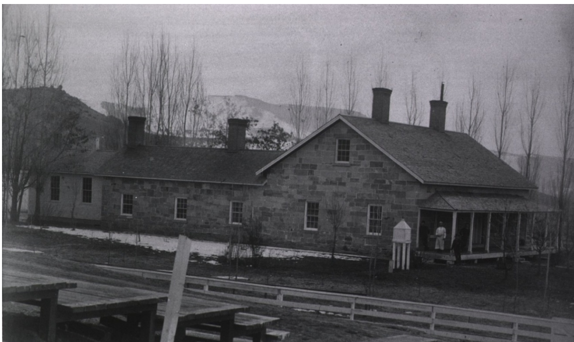
Figure 1. Boise Barracks Post Hospital with cotton region shelter (white) and rain gauge near porch. Date of Photograph: 1880 to 1895. Source: The History of Medicine (NLM), No. A01048.
