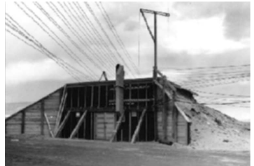
Fig. 4 – Trinity Site Main Bunker still exists today, minus the cables
