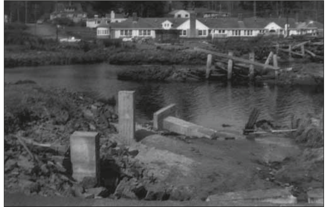
The tsunami generated by the 1964 Great Alaskan Earthquake (magnitude 9.2) caused over $250,000 dollars in damage and destroyed the Elk Creek Bridge in Cannon Beach.
