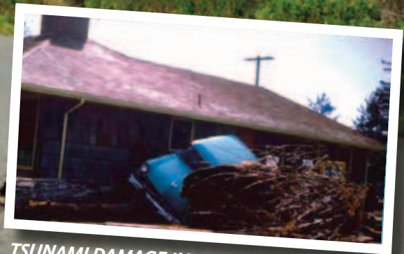
TSUNAMI DAMAGE IN SEASIDE FROM THE 1964 GREAT ALASKAN EARTHQUAKE
