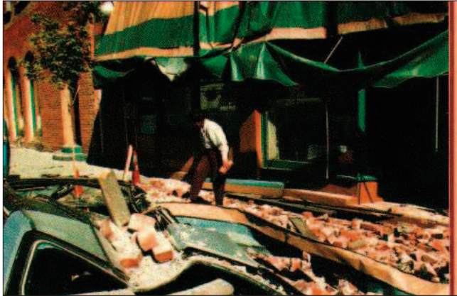
Downtown Klamath Falls after two magnitude 6.0 earthquakes in 1993. These were the largest earthquakes in history.
