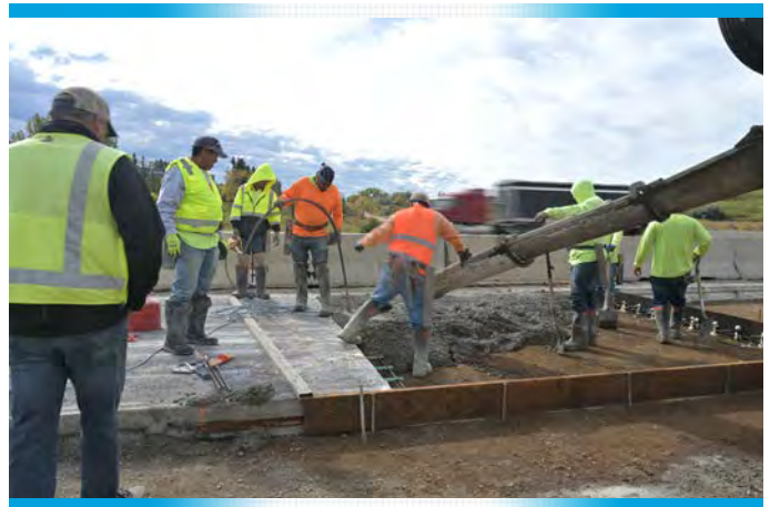
Paving on a slide repair project on I-94
