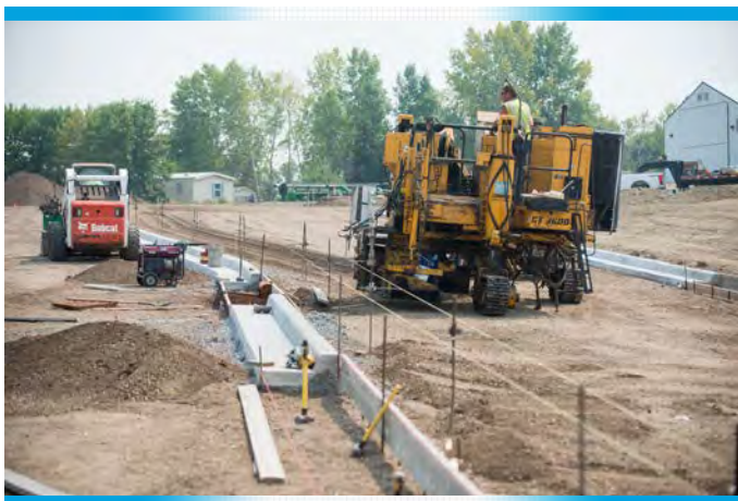
Installing curb and gutter on a project off of US 2
