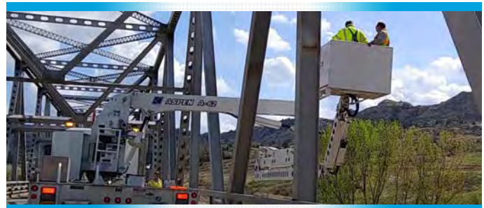
Bridge inspection on Long X Bridge
