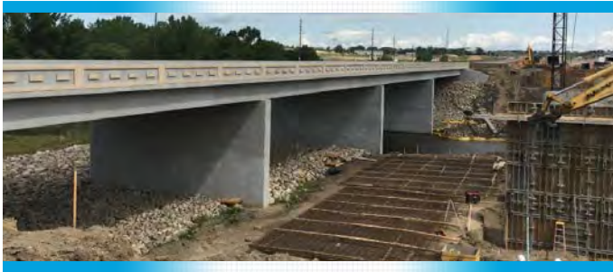
Construction of the US 83 Bypass in Minot
