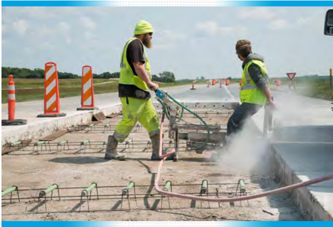
Concrete Pavement Repair (CPR) job on eastbound I-94
