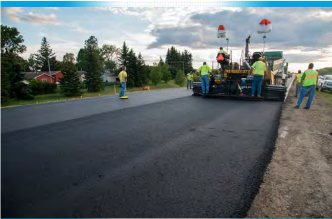
Asphalt paving of Interstate 94 through Bismarck District
