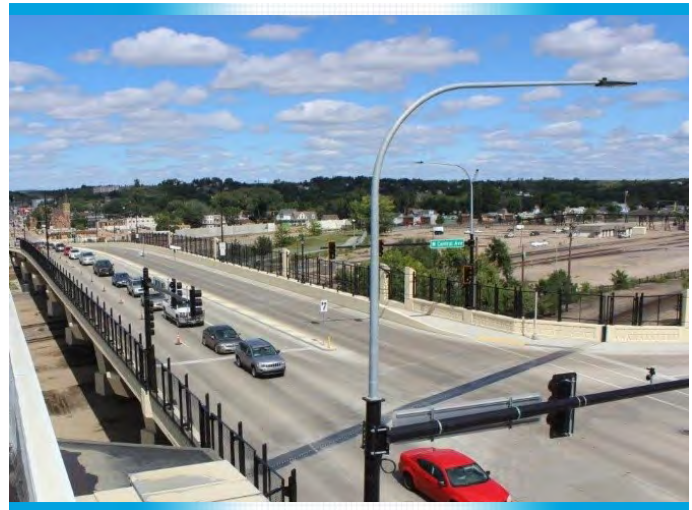
US 83 Broadway Bridge in Minot
