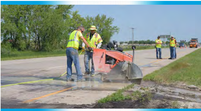
Concrete pavement repair on I-29 conducted by Grand Forks District employees
