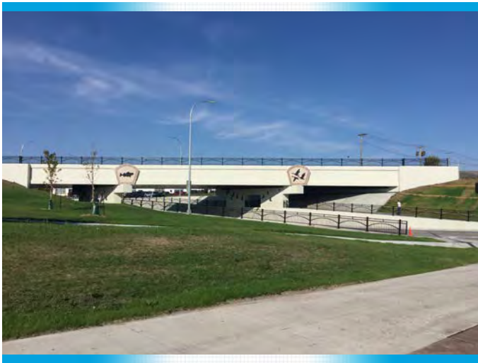
BNSF bridge in Devils Lake over ND 20
