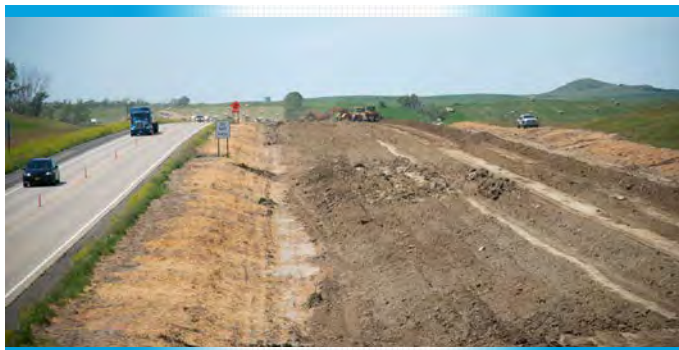
I-94 reconstruction project near Hebron
