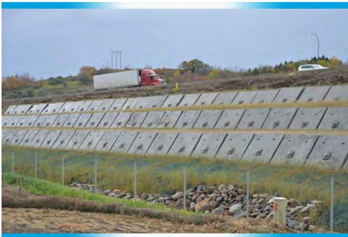
Ground anchors used to stabilize roadbed on I-94 through Valley City
