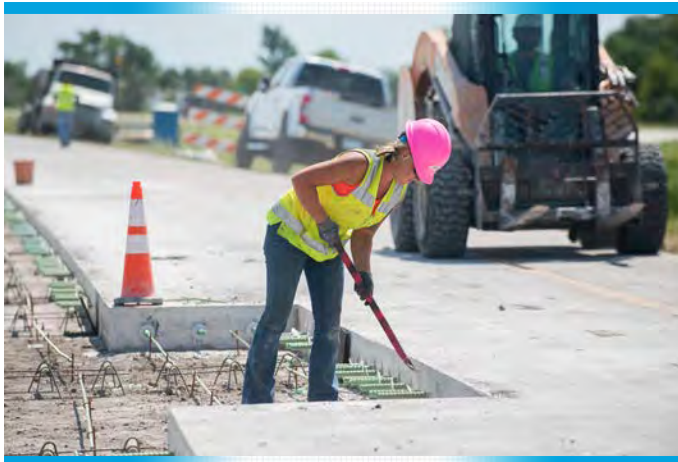
Moving ahead with a road projects in the Grand Forks District
