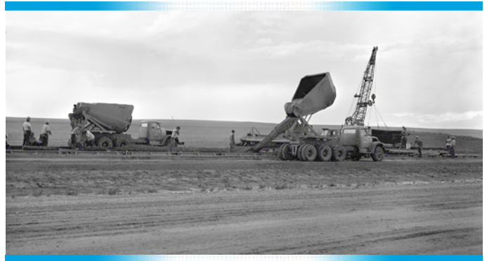
Concrete paving east of New Salem - 07-1963
