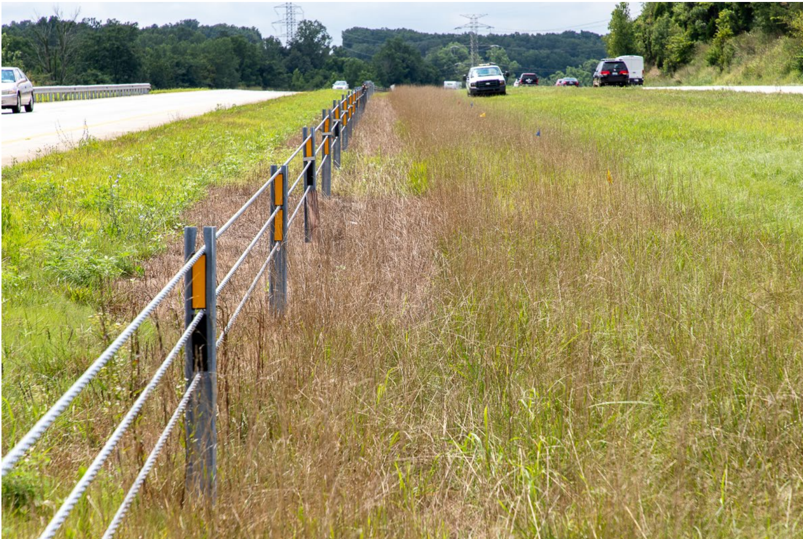
Figure 1: View of Plots in the Cable Barrier Trial on August 4, 2020 (63 Days After Treatment) Spray pattern observed on both sides of the cable barrier.
