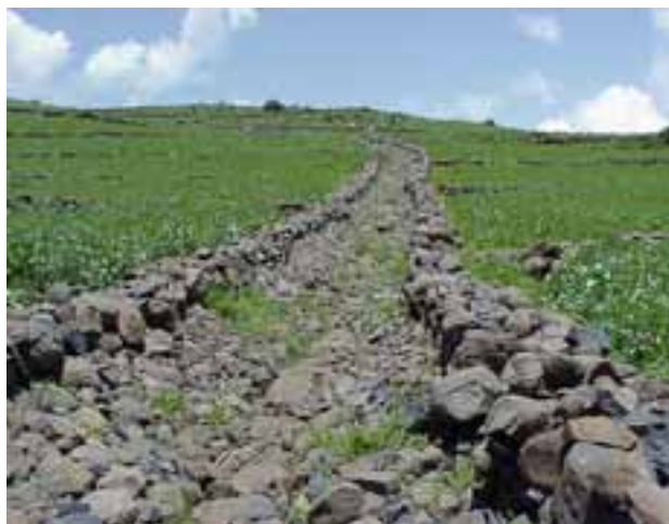
Graded terraces with paved waterways: high rainfall areas (all photos by Daniel Danano)
