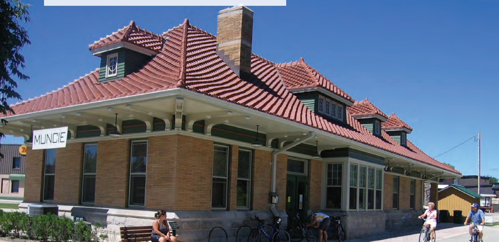
Rehabilitated passenger train station and Greenway trail in Muncie, Indiana
