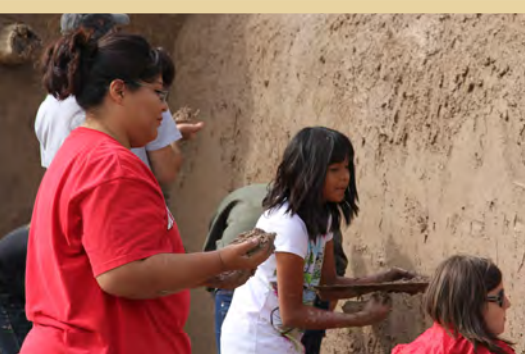
Mud plastering workshop at Ohkay Owingeh Pueblo, New Mexico (photo by Tania Hammidi)
