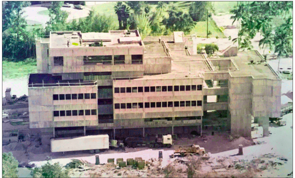
AOML under construction, circa September 1971. Photo credit: AOML archive.
