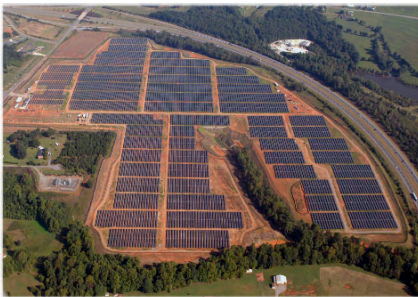
Maiden solar photovoltaic array
