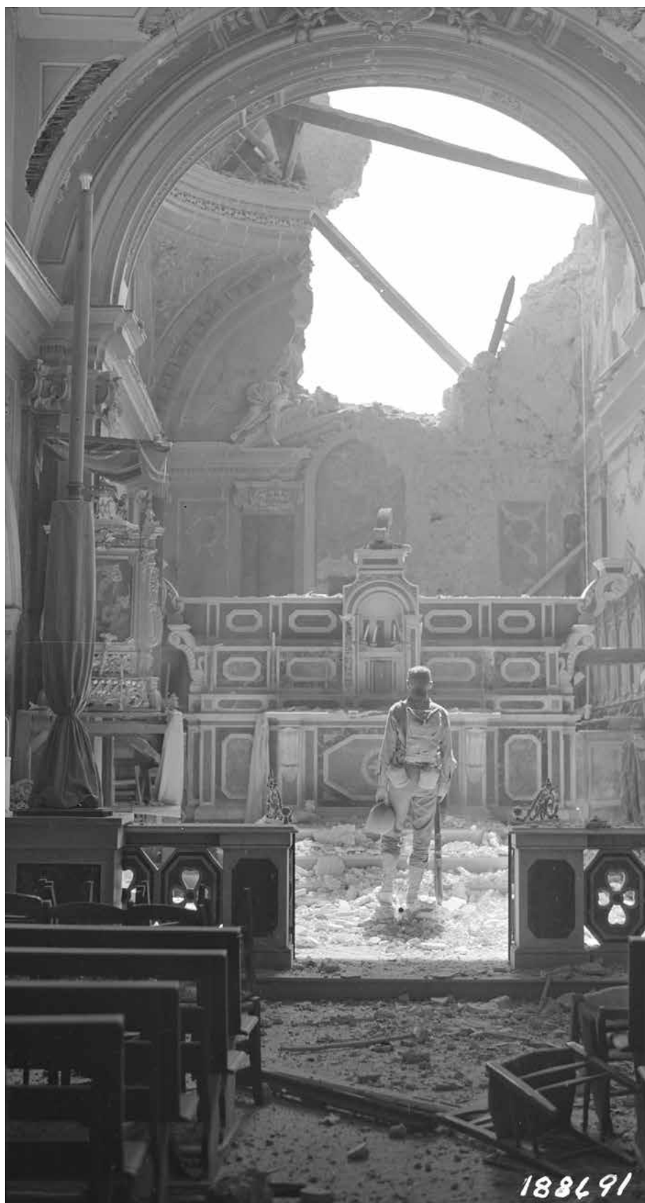
A damaged church in Acerno, Italy. Shipman and Jenkinson had visited churches, as many held vital local records.
