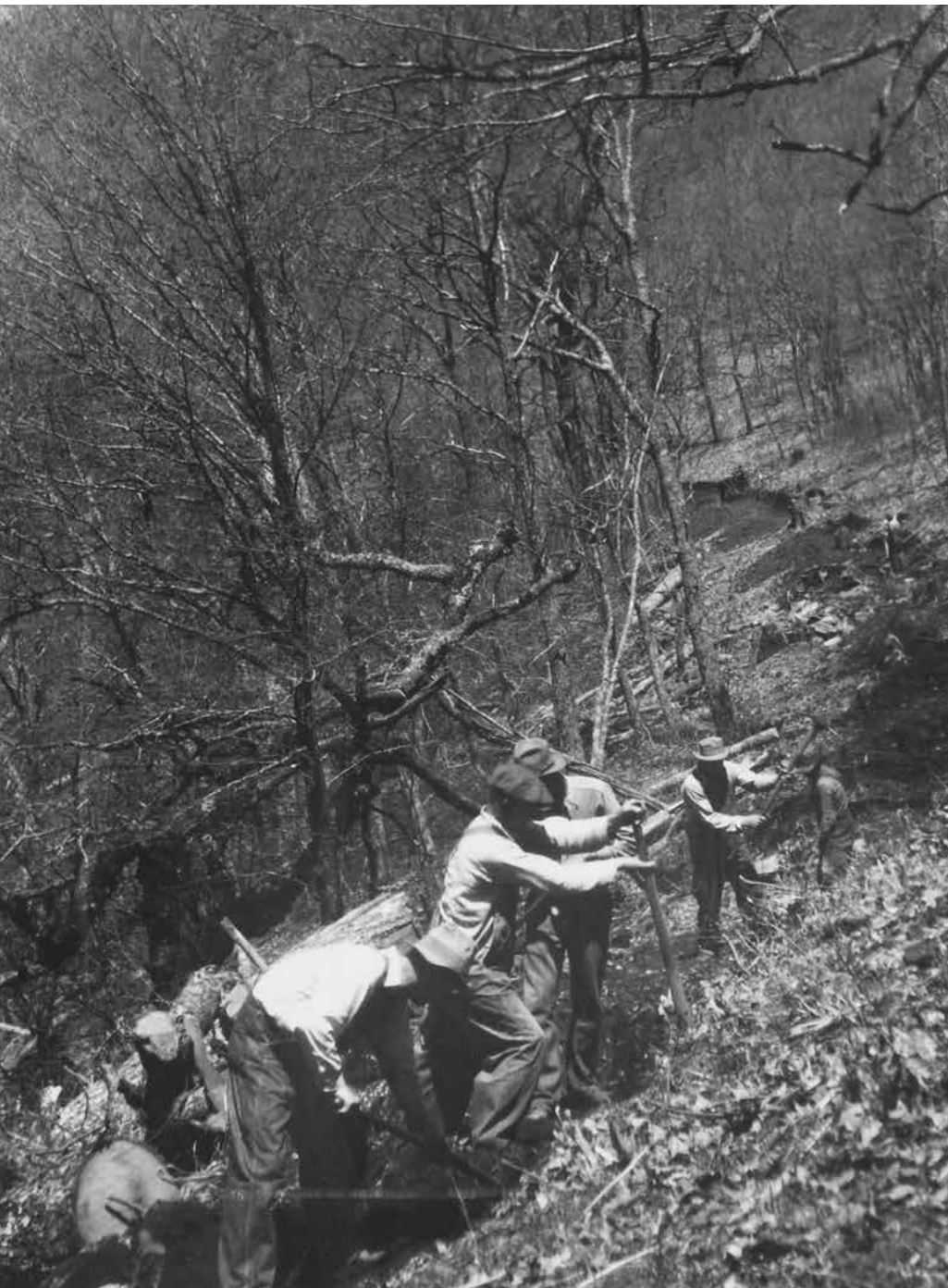
Left: Eastern Band workers breaking the Soco Gap truck trail. The trails and truck roads were largely cut by manual labor.
