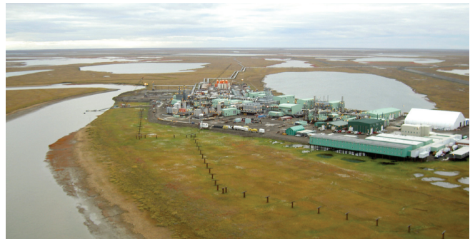
Figure 4.11. Alpine Oil Facility (ConocoPhillips Alaska) in Arctic Alaska. (Photo credit: D. White)
