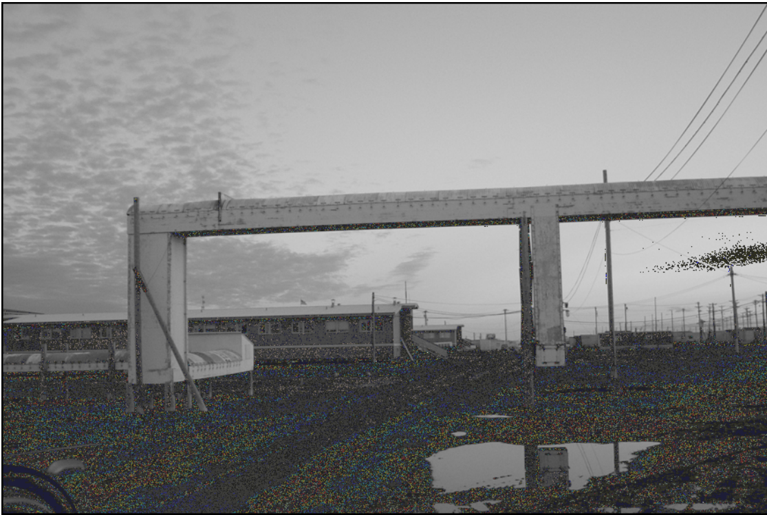
Figure 9. Utilidor in Barrow, Alaska.
