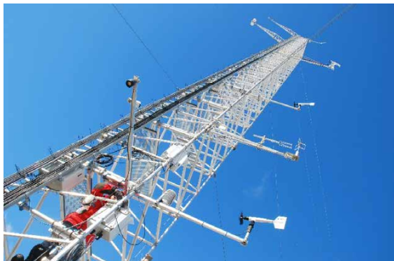
The Amundsen-Nobile Climate Change Tower during maintenance. Photo: Fabio Giardi, University of Firenze
