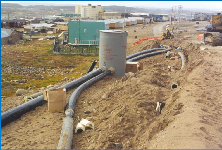
Water and sewer replacement in Iqaluit, NU in 1995.
