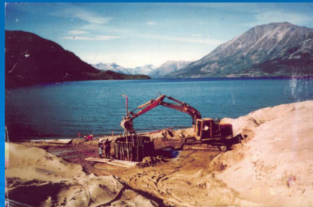
Water intake construction in Carcross, YT in 1990
