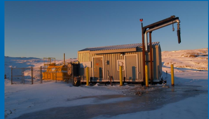
Water treatment facility Kimmirut, NU
