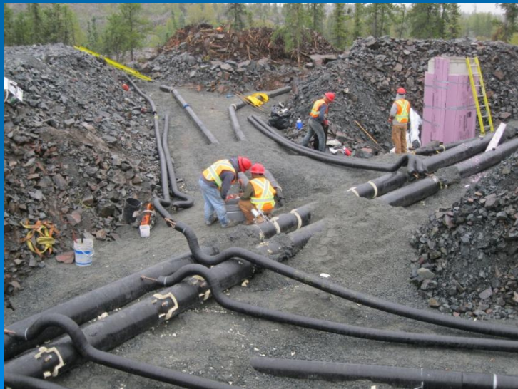
Water and sewer replacement in Yellowknife, NT in 2011.
