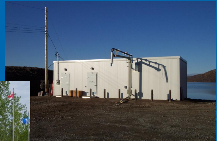
Water treatment facility for Ulukhaktok, NT – on route and in place
