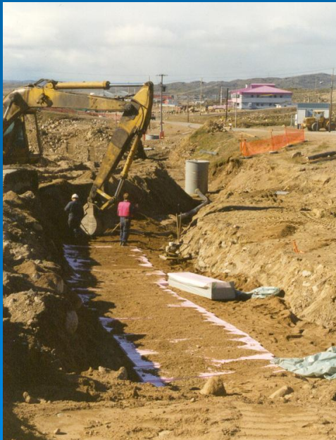
Buried water and sewer system in Iqaluit, which will be similar to the Resolute system
