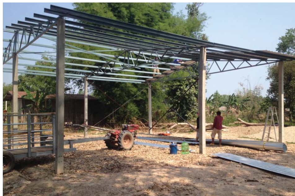
A harvest center under construction.
