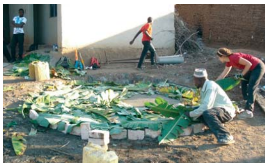
Building a brick-and-mortar water tank (left to right): UMN student Danielle Chase and community member Yasin cover the foundation with banana leaves while it cures, the tank under construction, and the finished tank with cover installed.
