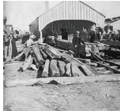
Figure 8.2. Burnettizer in operation c.1863. Vacuum chamber entrance is on left side. From: S.E. Ambrose, “Nothing Like it in the World - The Men Who Built the Transcontinental Railroad 1863-1869” (Touchstone Pub., New York, 2000).
