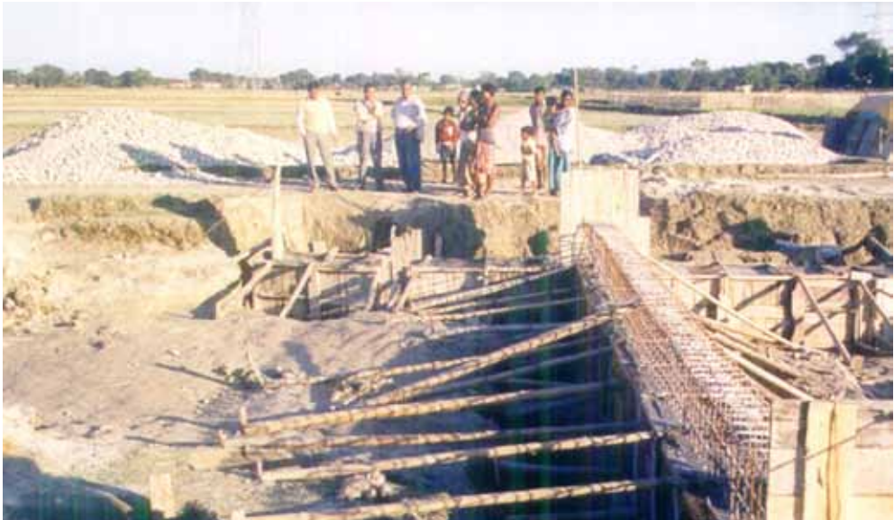
Figure 2: Constructing a gully plug to retain groundwater
