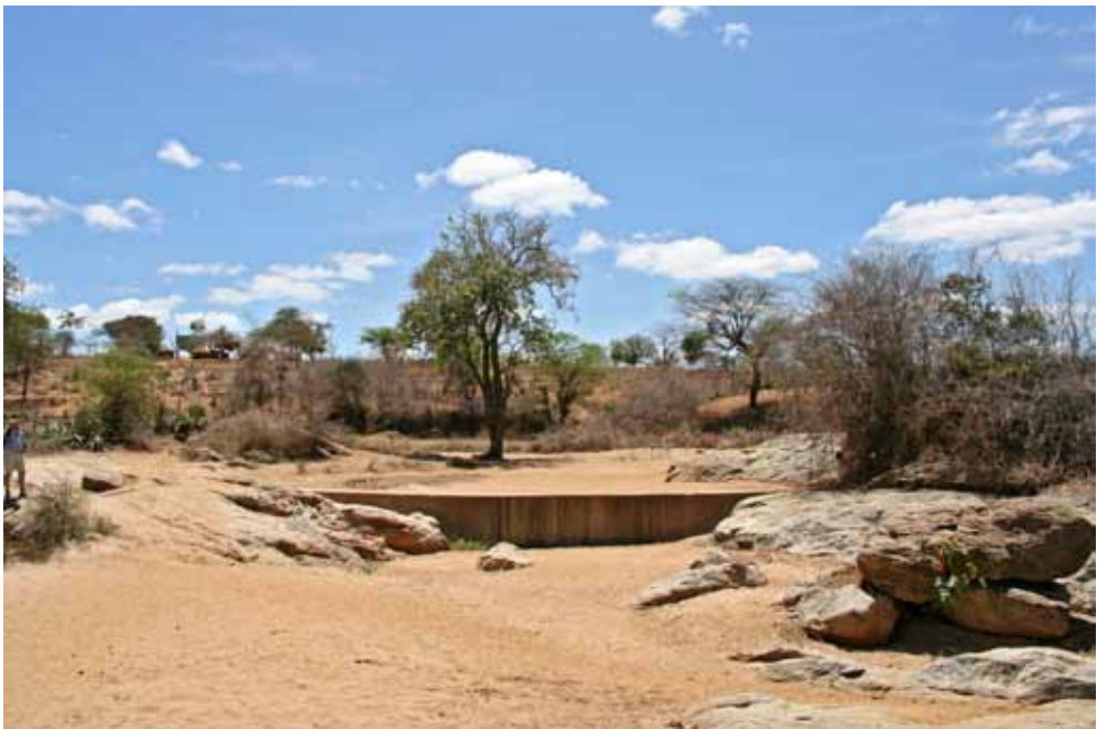
Figure 1: A typical sand storage dam during the dry season in the Kitui District
