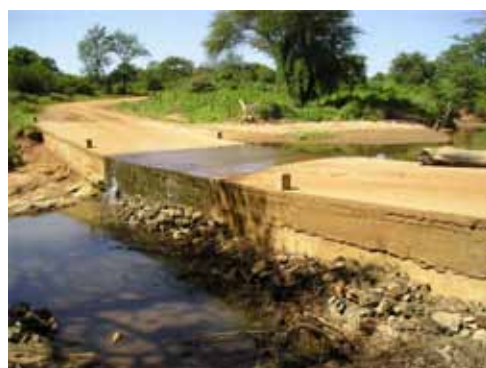
Figure 3: Irish bridge (Source: Nissen-Petersen, E, 2006)
