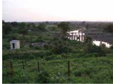
Figure 2: River bank infiltration well in Maharashtra
