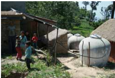
Figure 1: Rainwater harvesting tanks in Bubeyrakhe, Nepal
