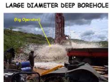
Figure 4: Drilling of large diameter deep borehole
