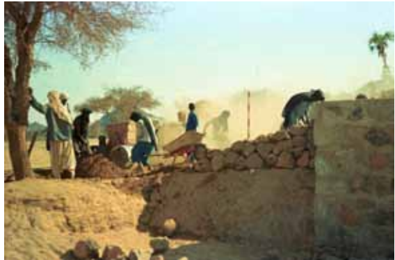
Figure 2: Construction of diversion works
