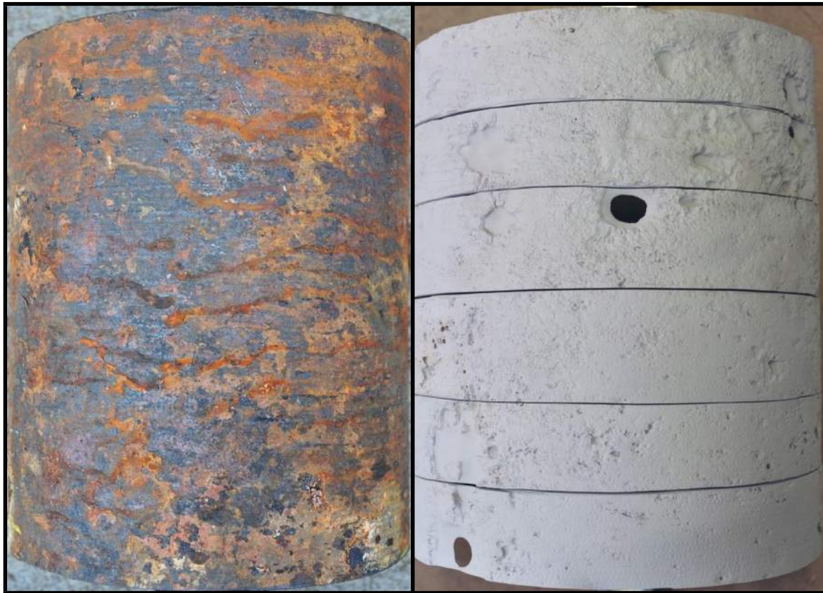
Figure 11-6 Excavated Pipe Showing Graphitic Corrosion Before (left) and After (right) Sandblasting
