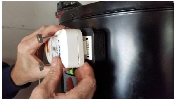
Figure E-1. Wireless Communication Hardware Getting Connected to the CTA-2045 Port on a Water Heater
