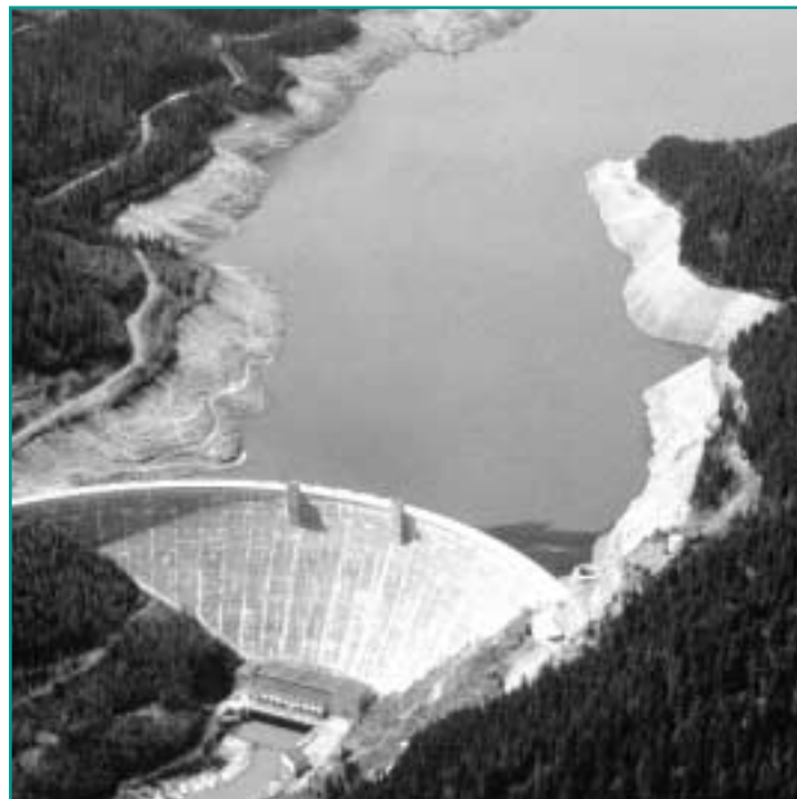
Hungry Horse Dam is an important component of the region's power generation system, turning water into kilowatts of electricity.
