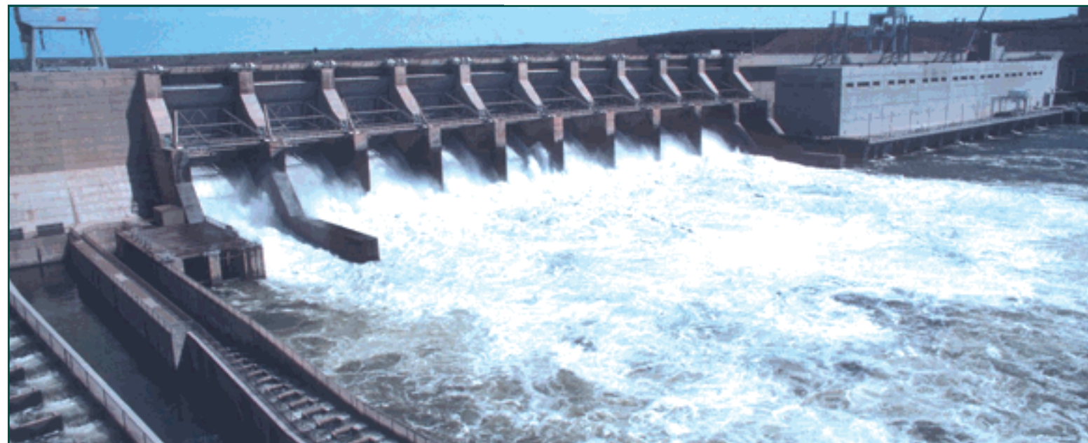
Ice Harbor Dam
