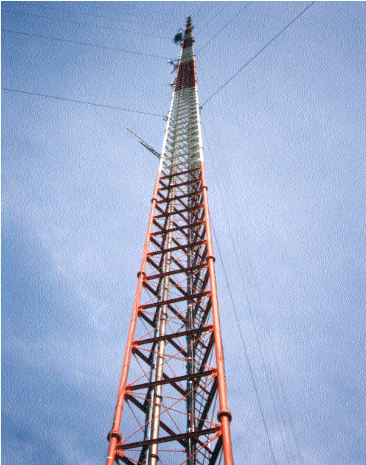
Photograph of the 447-meter tall WLEF-TV transmitter tower, Park Falls, Wisconsin. The tower is owned by the State of Wisconsin Educational Communications Board, and is being used for measurements of CO 2 mixing ratios (see Bakwin et al., 1998) and atmosphere/surface exchange of CO 2 by eddy covariance. Transmitter towers up to 610 meters tall are located in many areas of the USA.
