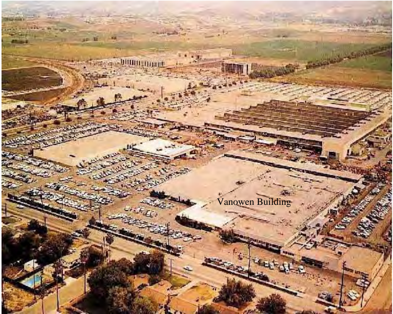
Figure 5-1: The Canoga Park Facility in 1960
