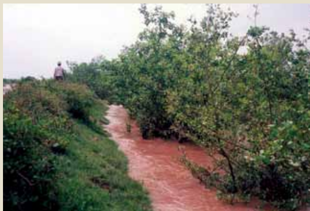
Figure 20: The use of mangroves in hybrid structures to reduce risk from storm surge flooding in Vietnam; here mangroves reduce the energy of wind waves reaching the dike, reducing the likelihood of damage to the dike or of waves overtopping it. Credit: Mai Sỹ Tuấn (used with permission)
