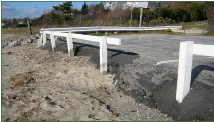
Pictures of Barrington Beach— (Top left) Before: erosion is evident at the western end of the parking area. (Top right) After: the parking lot is reduced in width and beach grass planted. (Right) After: Parking lot pavement removed, beach grass planted. This project also included the installation of stormwater infiltration practices to address runoff from the adjacent streets. (Photos courtesy of Save The Bay)
