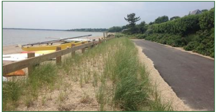
Pictures of Barrington Beach— (Top left) Before: erosion is evident at the western end of the parking area. (Top right) After: the parking lot is reduced in width and beach grass planted. (Right) After: Parking lot pavement removed, beach grass planted. This project also included the installation of stormwater infiltration practices to address runoff from the adjacent streets. (Photos courtesy of Save The Bay)
