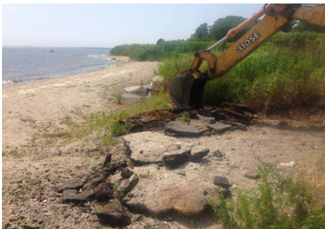
Van Zandt Avenue, Warwick. An end of road adaptation project completed in 2017 removed eroded pavement and installed a filter strip. (Photo: CRMC, Save The Bay)
