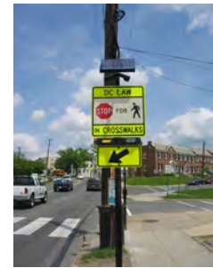
RFB at Brentwood Rd. NE, Washington, DC
