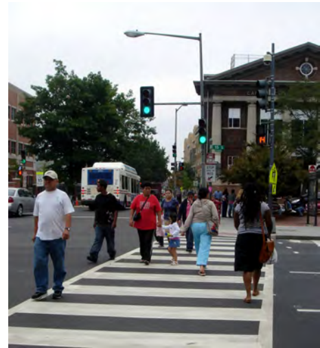
High visibility crosswalk markings on 16 th Street, NW.
