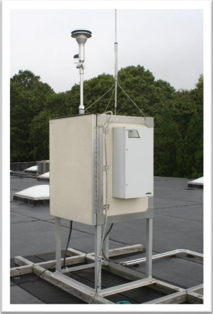
Figure 13: Narragansett Monitoring Shelter
