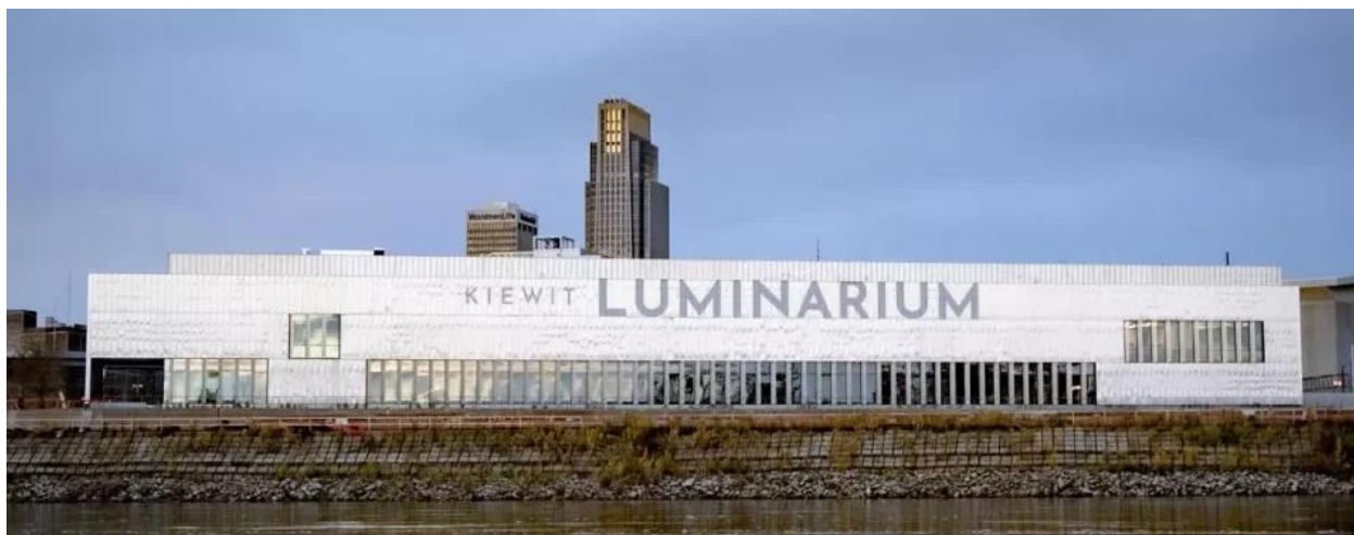
The photos on the top row show cleanup activities at the Lewis and Clark Landing Kiewit Discovery Center Foundation in Omaha. Remedial measures were taken during construction of the foundation of the Kiewit Luminarium to address and repair disturbances to the multi-layered protective capping system that was installed during cleanup of the American Smelting and Refining Company site (photos courtesy of the Remedial Action Report dated October 20, 2021). The photo on the bottom row shows the completed Kiewit Luminarium, which opened to the public on April 15, 2023, as a community space and interactive learning environment (photo modified from the Kiewit Luminarium webpage).
