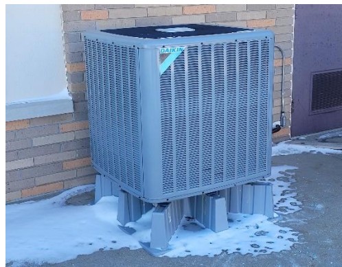
Left: A 7.2 kW Residential Photovoltaic system, Lincoln (2022); Right: A 5 ton, 16 SEER AC unit, part of a $320K HVAC project for Broken Bow United Methodist Church, Broken Bow (2022).
