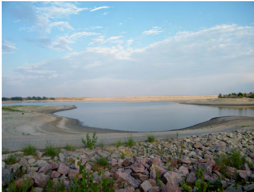
Davis Creek Reservoir, Valley County, looking toward dam. 2012 drought impact: water level down ~ 25 feet.
