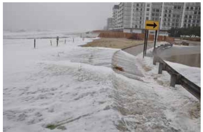
Surf Avenue in Rehoboth Beach floods during Hurricane Sandy. In Sussex County, between 27 and 39 miles of evacuation routes could be underwater with a sea-level rise of 1 to 1.5 meters. Photo: Delaware Sea Grant/University of Delaware
