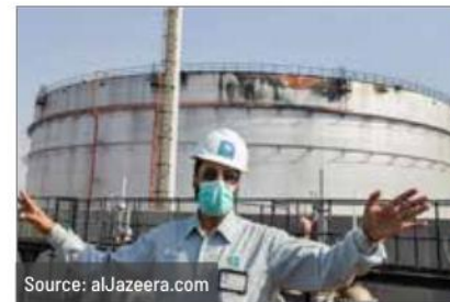
A Saudi Aramco oil silo in Jeddah, Saudi Arabia, damaged by a Houthi missile attack in November 2020 47
